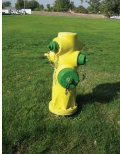
Wet barrel hydrant (warm climates)
