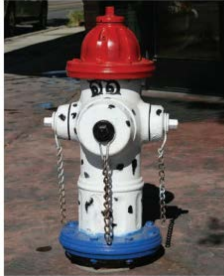
Dry barrel hydrant (freezing temperatures)
